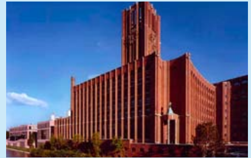
9 Deutsche Bank Communication Center in the historic Ullsteinhaus in the Berlin district of Tempelhof
