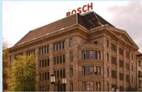
8 Bosch Communication Center Germany in the Berlin district of Charlottenburg
